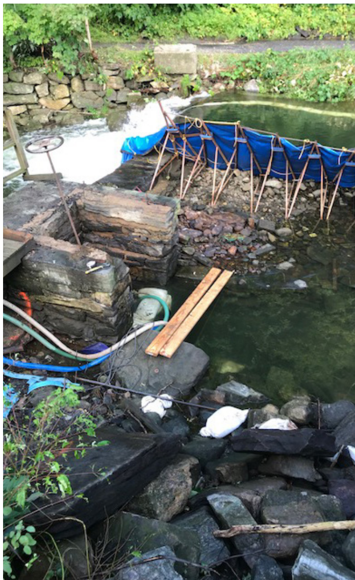
Dam construction (gate valve replacement)
