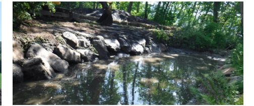
Basin After Clean Out
