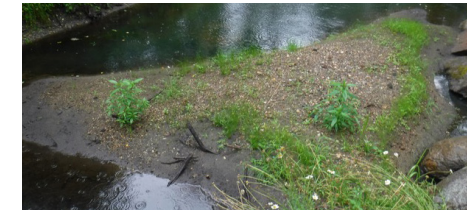
Basin Before Clean Out
